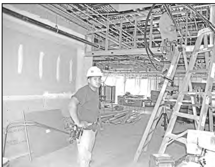
Work has begun on the media center that will swap places with the guidance suite.
