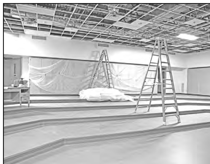
Renovations are underway in the bandroom at William Byrd.
