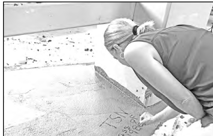
Principal Tammy Newcomb, a William Byrd graduate, leaves her initials and graduation year in the newly poured concrete – which will be covered during renovations.
