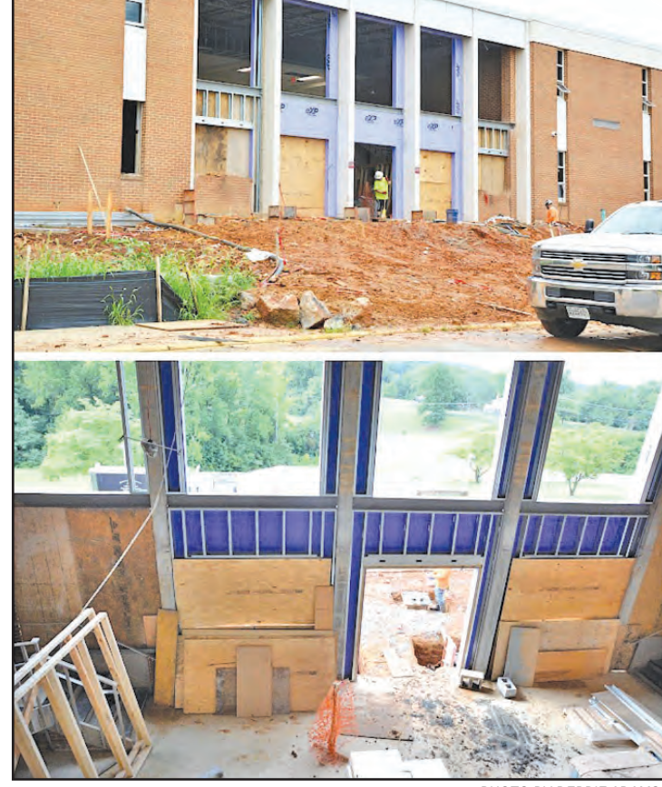
PHOTO BY DEBBIE ADAMS Renovations are being made to the front entrance and front lobby of Byrd.
