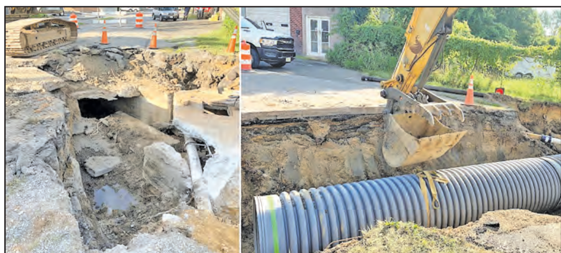
The project Vinton Public Works completed on North Maple Street.
