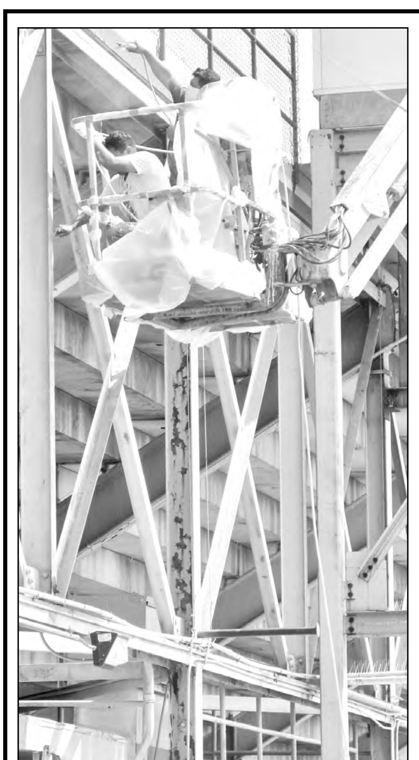
William Byrd's Patterson Stadium recently got a fresh coat of paint. Here workers spruce up the stadium.
