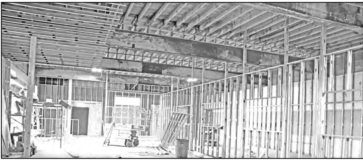
The interior of the new Pollard 107 South restaurant has been completely gutted for renovations.
