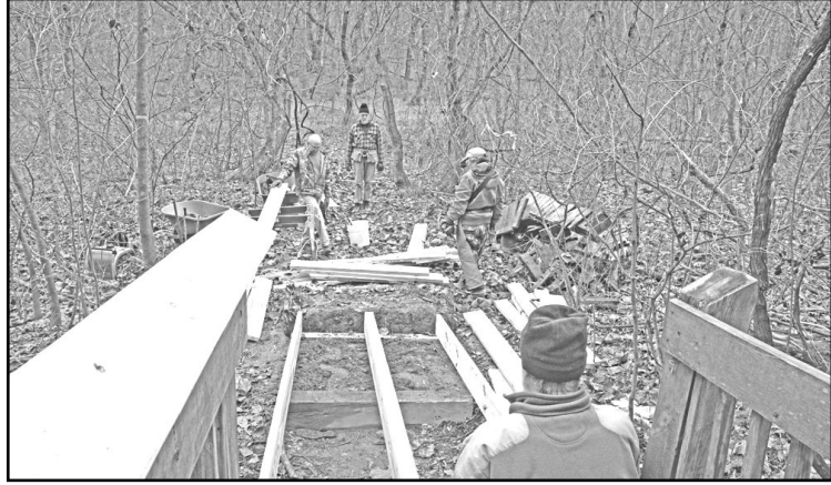
Gladetown Bridge repair —2022. PHOTOS BY DEBBIE ADAMS
