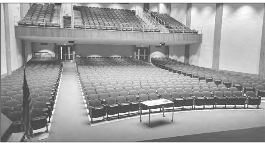
Renovations are substantially complete to the WBHS auditorium.
