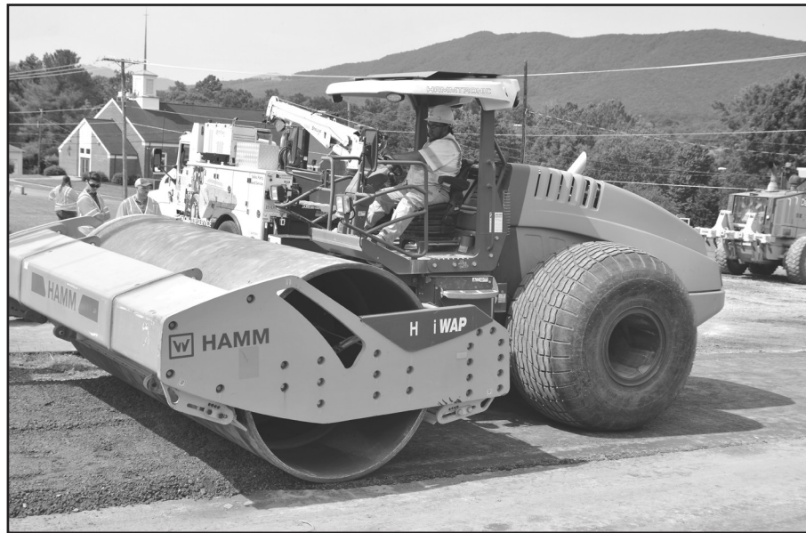
A powerful roller is used to compact the base material.
