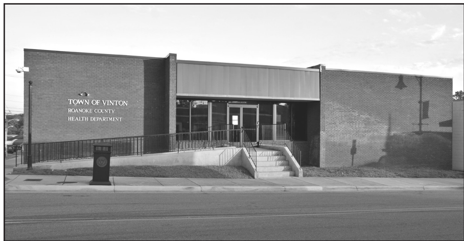
The upper level of the Roanoke County/Vinton Health Department on Pollard Street has been renovated and now serves as the town Annex.
