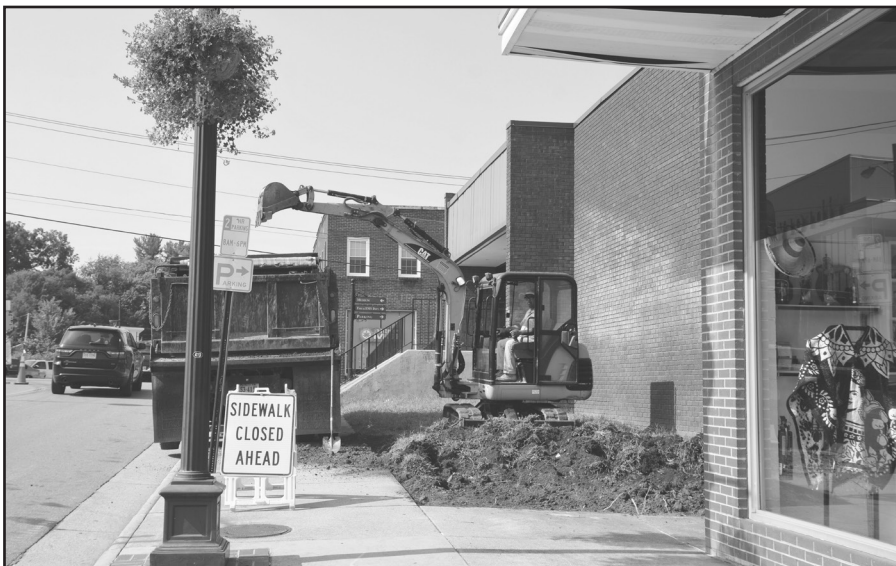
Work is underway on landscaping/hardscaping at the Town of Vinton Annex.
