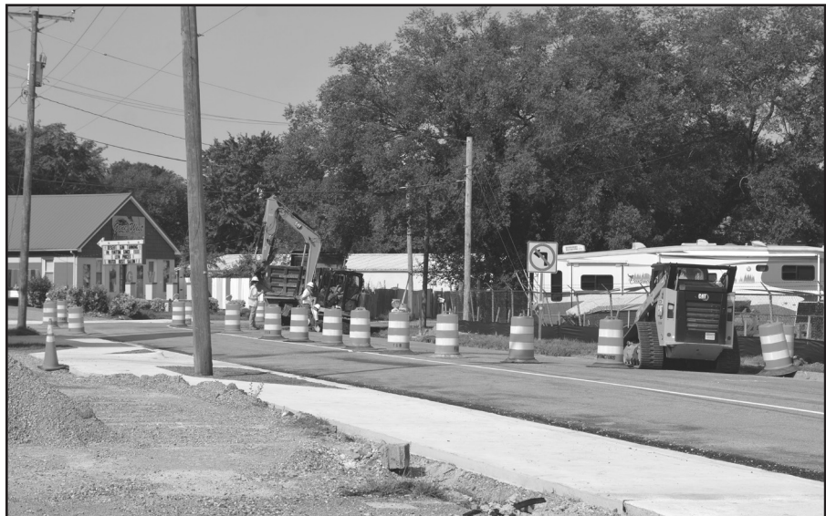
Construction continues on Walnut Avenue.
