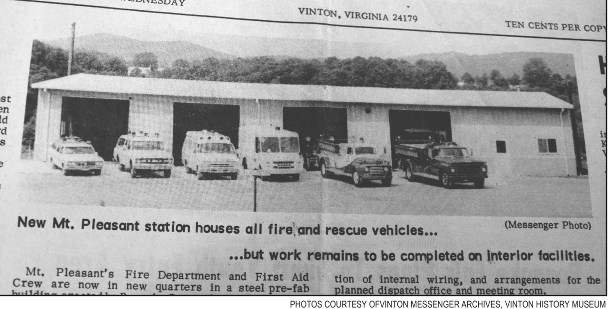
The Mt. Pleasant Fire Dept. and First Aid Crew moved into new quarters—a steel pre-fab building erected by Roanoke County.
