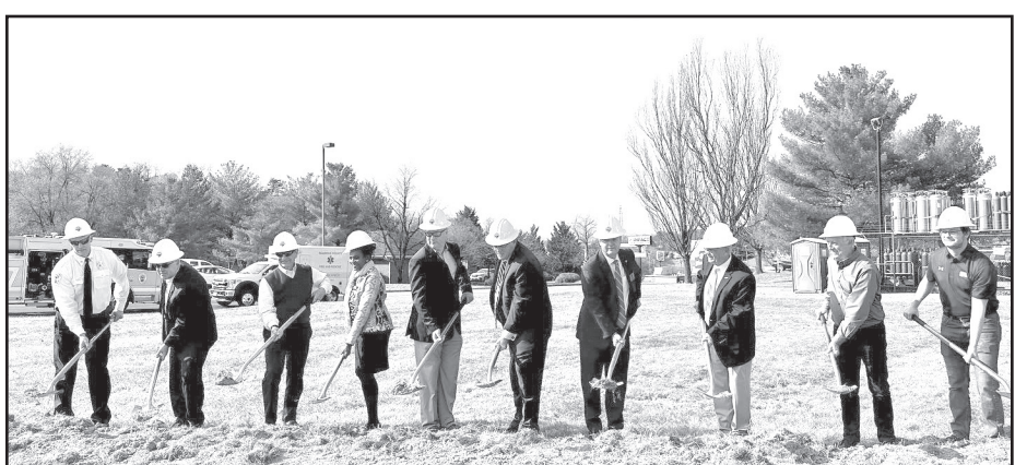
A groundbreaking was held for the new fire and rescue building in Bonsack on Nov. 16.
