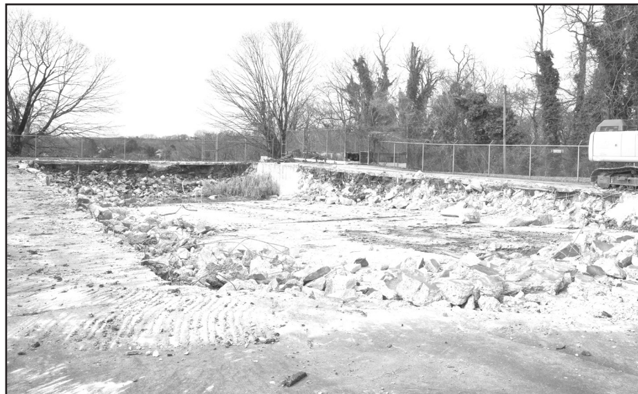
Lee Lovern is the contractor for the demolition phase.
