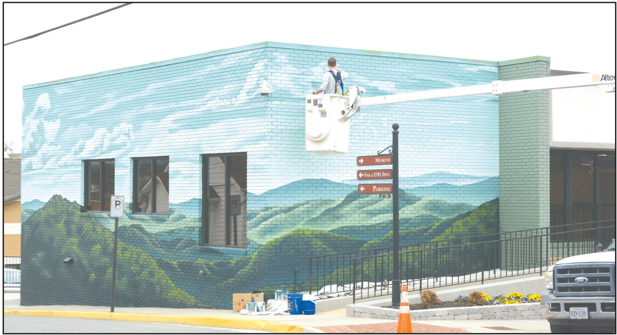
Jon Murrill is in his second week of work on the Lady Appalachia outdoor mural in downtown Vinton, on some occasions using a bucket truck, rather than a ladder, to reach the tops of the wall at the Town of Vinton Annex on Pollard Street. Plans are to complete the project in early April.
