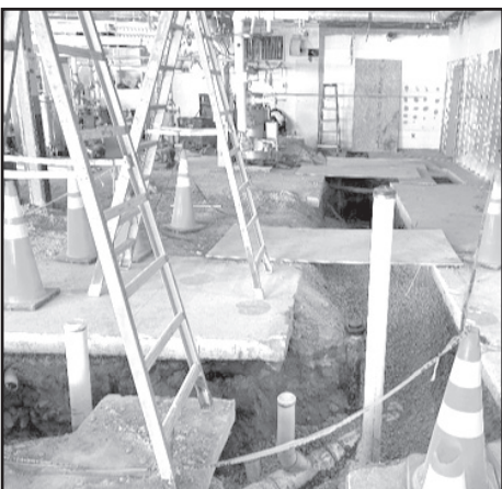
Floors have been cut for plumbing at the W.E. Cundiff renovation project.
