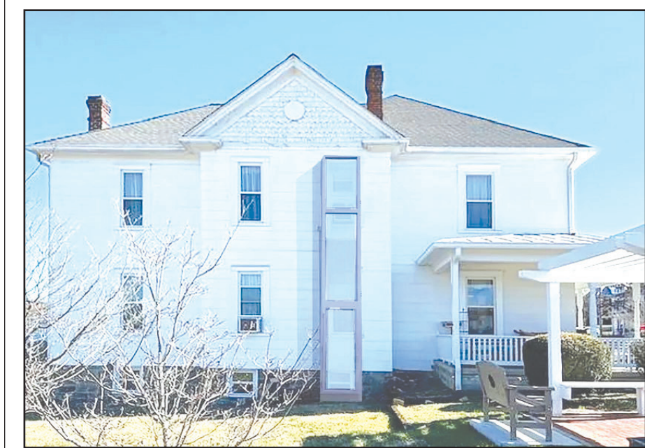
Rendering of the ADA lift to be installed at the Vinton History Museum. PHOTO COURTESY OF VINTON HISTORY MUSEUM
