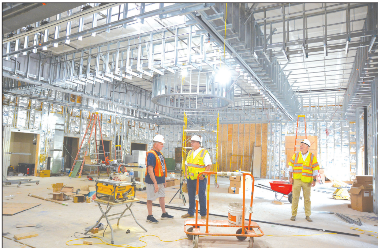
Council member Mike Stovall, Capital Projects Director Jamie Hurt, and Town Manager Pete Peters led a renovations tour of the Vinton War Memorial before the walls are closed up. An enormous light fixture and the bulkhead the ceiling will attach to are still visible.
