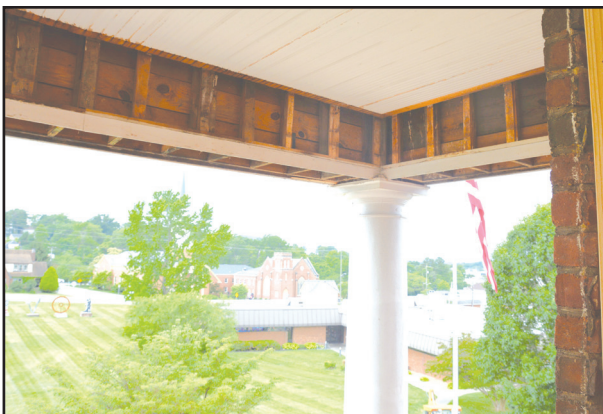
The original portico roof at the Vinton War Memorial
