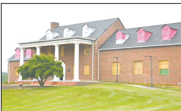
The Vinton War Memorial is undergoing extensive renovations, mainly in the interior of the building.
