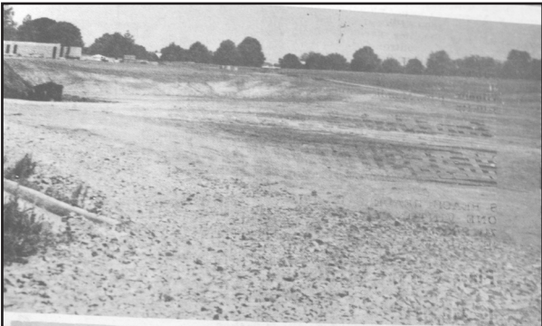
A photo of a grading site in 1976 for construction of Berkshire Nursing Home
