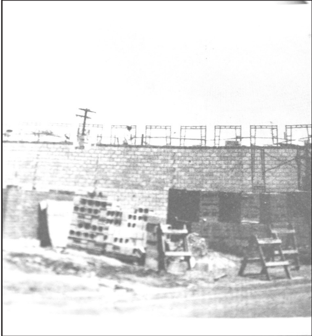
New Vinton Fire Station under construction in 1976
