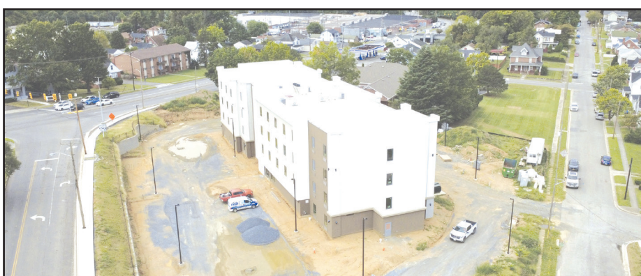
Drone photograph of Vinton Hotel
