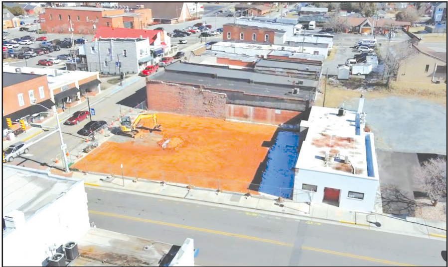
Downtown Vinton property site ready for development
