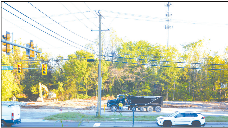
Demolition was begun and completed within about a week at the former Rite Aid location on Hardy Road.
