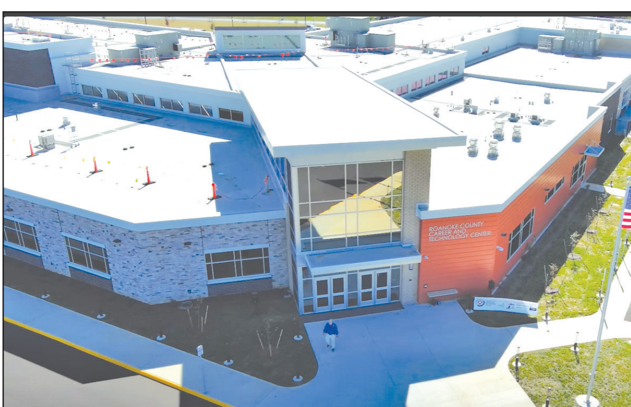
The new Roanoke County Career and Technology Center campus off of Peters Creek Road
