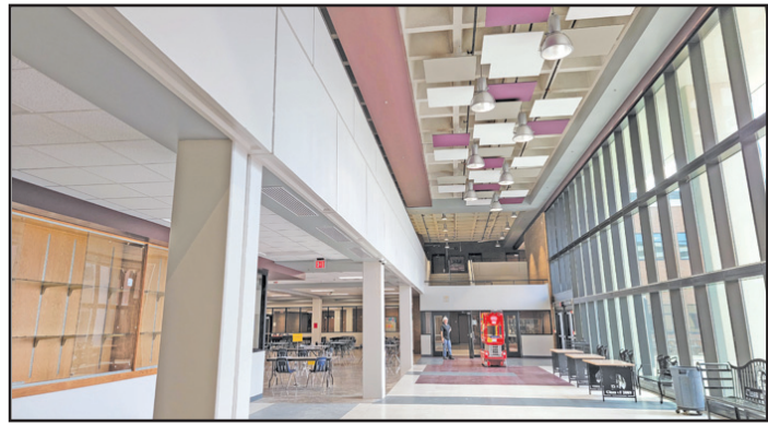
This "cloud system" architecture ceiling is in place above the old cafeteria space.
