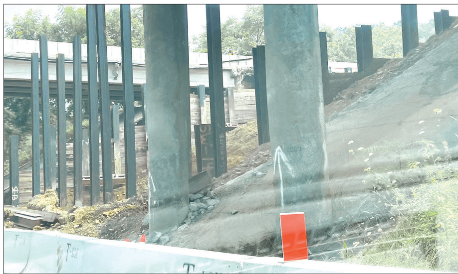
The repairs involved removing damaged concrete, replacing reinforcing steel and pouring new concrete.
