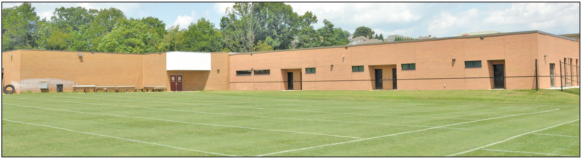
Above, doors to the Salem High fieldhouse open to a lush practice field that was once the Salem High baseball field. The former fieldhouse, for football only, is at the left of the white overhang.
