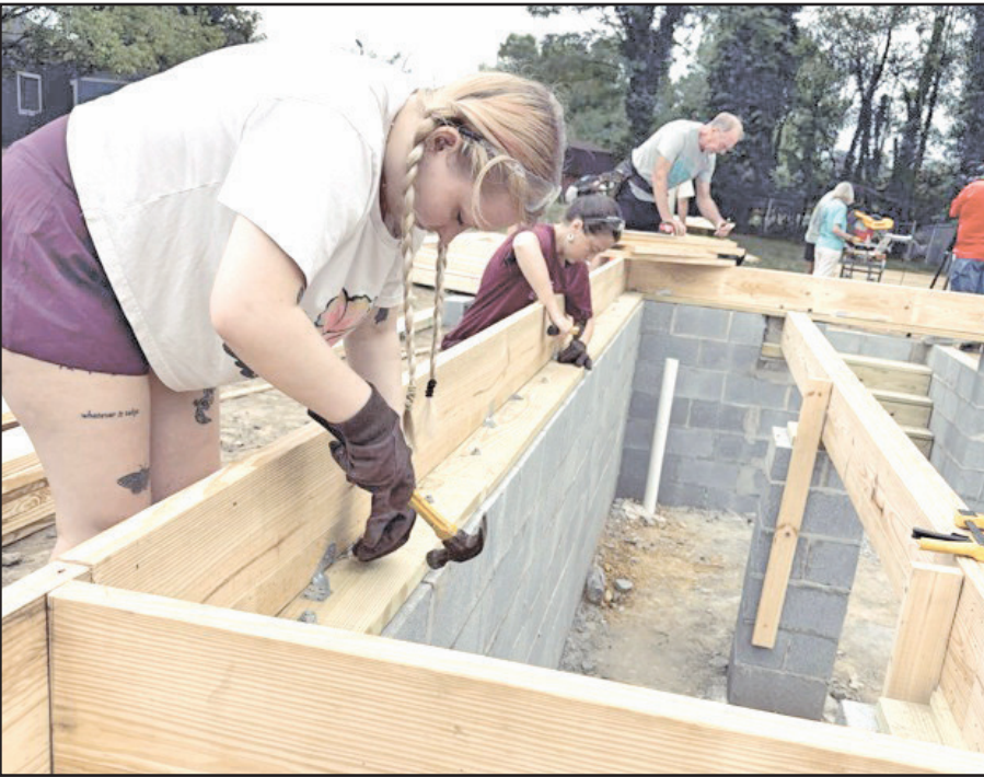
Construction started on Friday.
