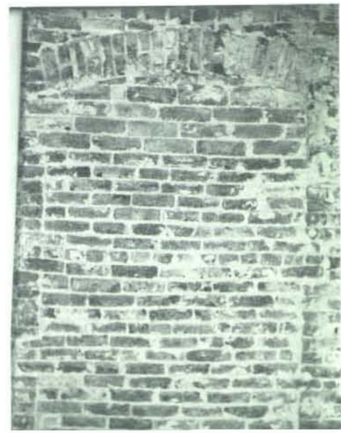
FIG. 5. Bricked up doorway, with arch support, between side hall and southwest bedroom which will be opened and fitted with proper woodwork.
