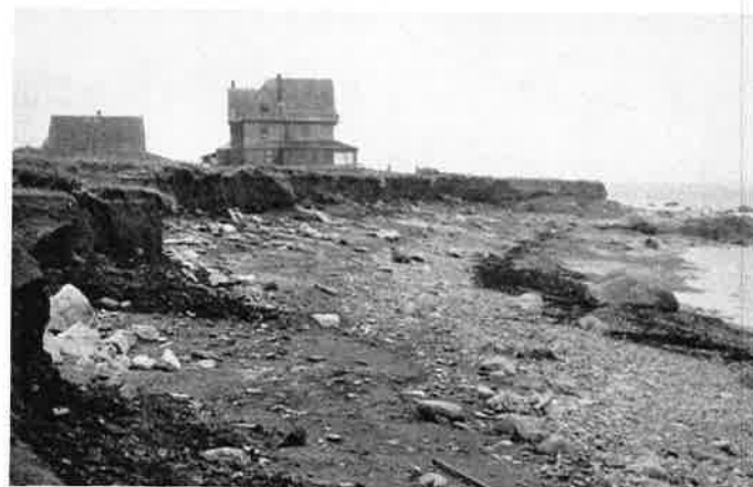
FIG. 16 (above)—Warwick Point Light, nearly undermined by 38-foot erosion of glacial debris and hard pan on a bench of graphitic shale flush with the five-foot bulkhead.
