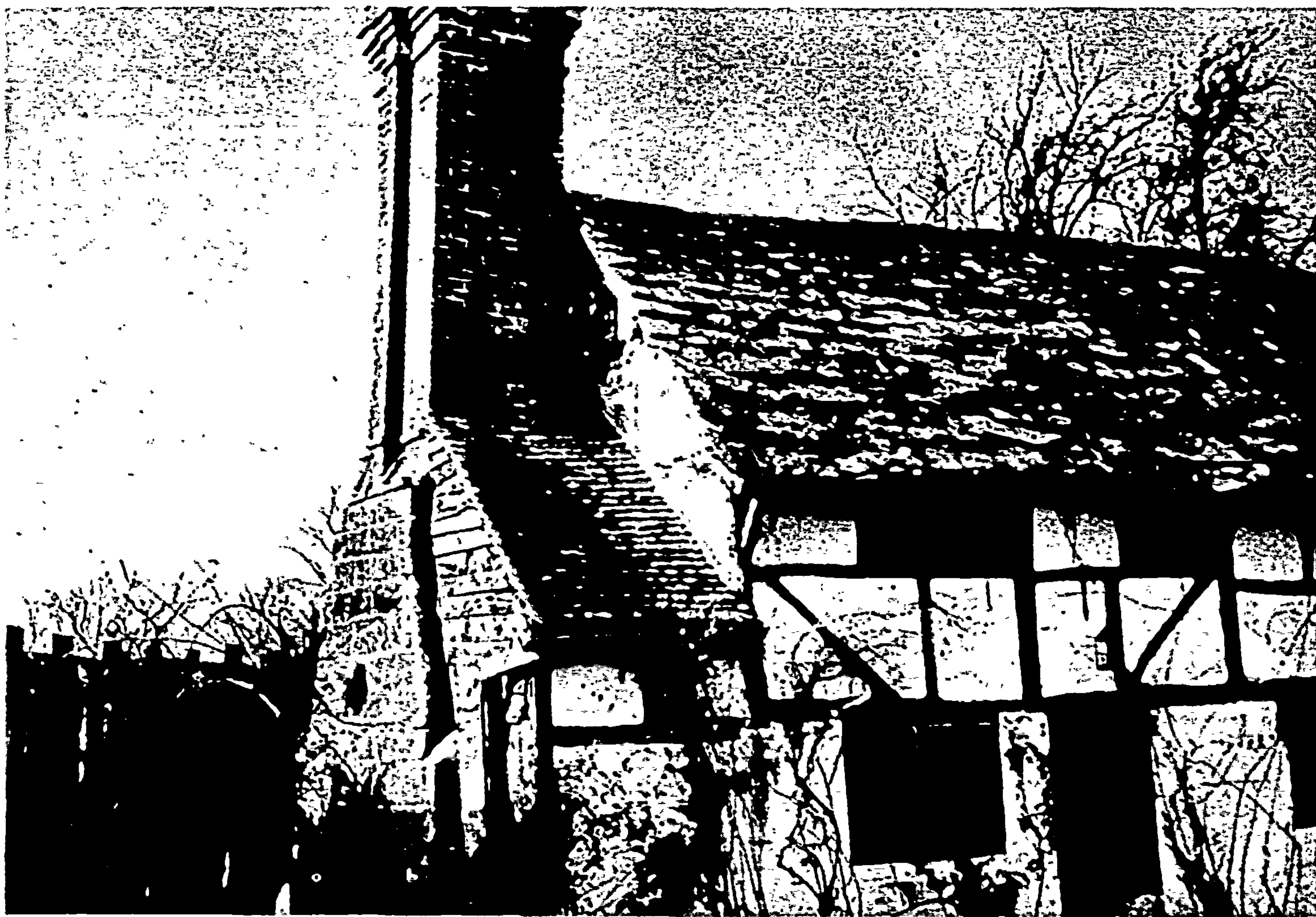
↑ PILASTERED chimney stacks, projecting caps show relationship between Eleazer Arnold house (above), Great Road, Saylesville, built 1687, and Badger's Cottage, Wineham, Sussex (below) built in 15th century. Original Arnold lean-to followed the chimney pitch (left). ↓
