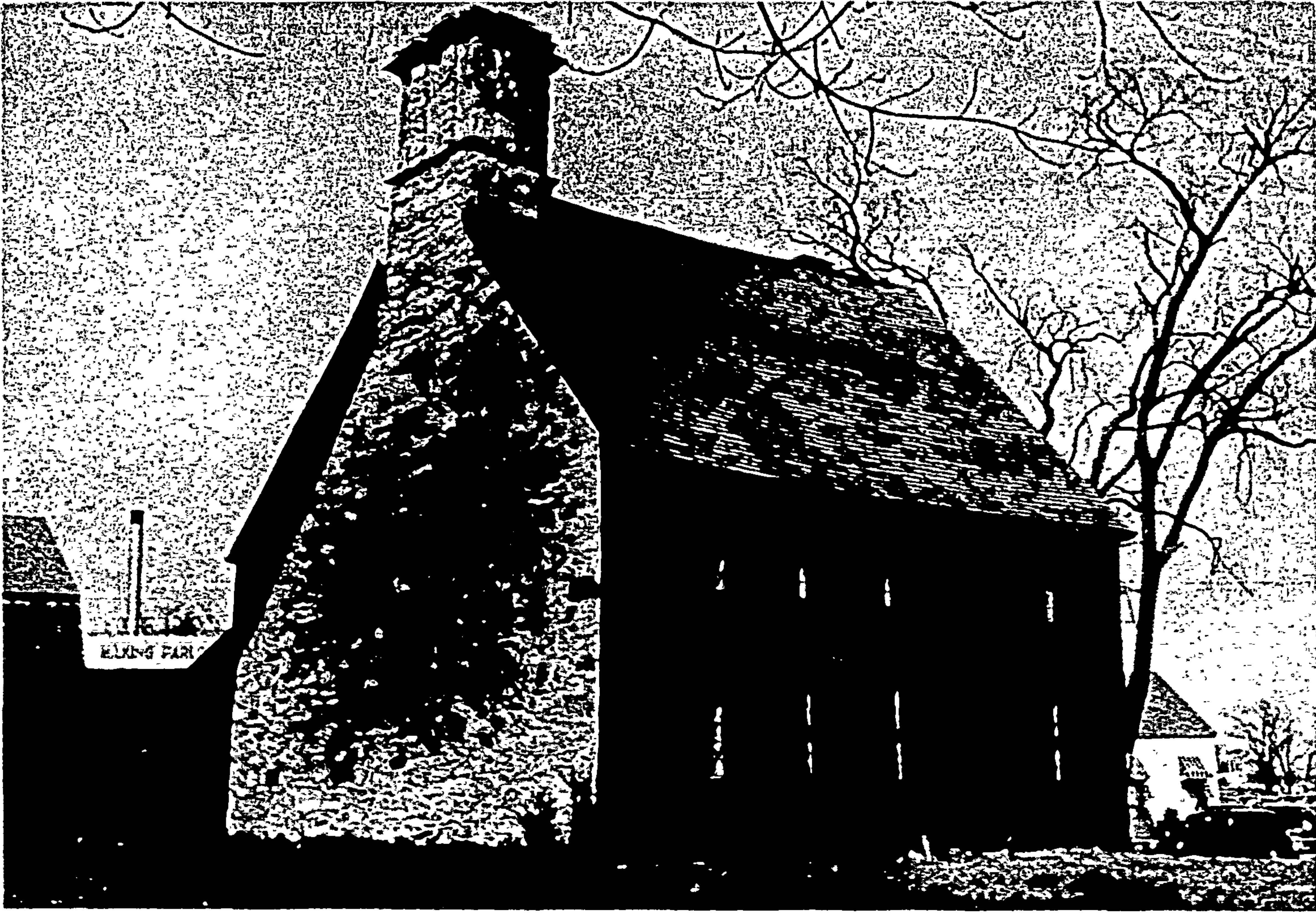
↑ PILASTERED chimney stacks, projecting caps show relationship between Eleazer Arnold house (above), Great Road, Saylesville, built 1687, and Badger's Cottage, Wineham, Sussex (below) built in 15th century. Original Arnold lean-to followed the chimney pitch (left). ↓
