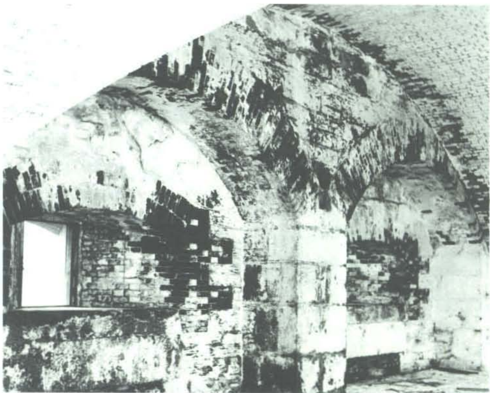
Fig. 14. View of casemate arches and embrasures.
