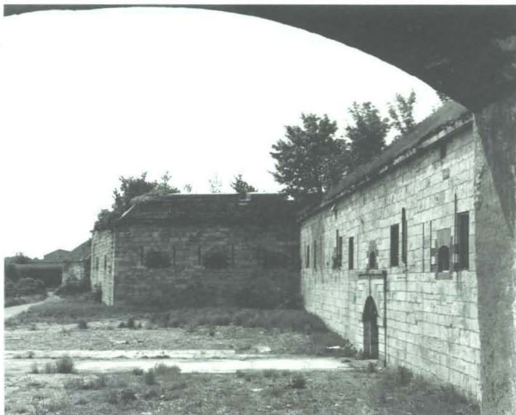
Fig. 7. View of southeast demibastions from fight flank of northeast bastion.
