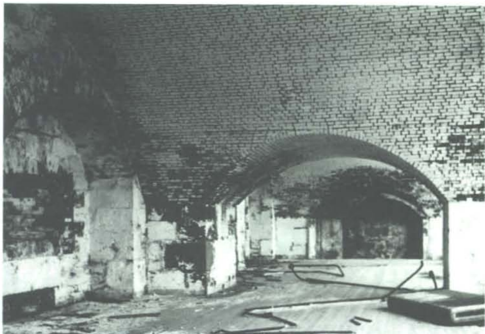
Fig. 13. Second tier of casemates on west front.
