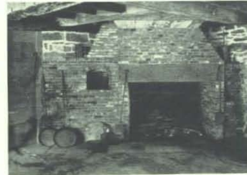
FIRE PLACE, GILBERT STUART HOUSE
