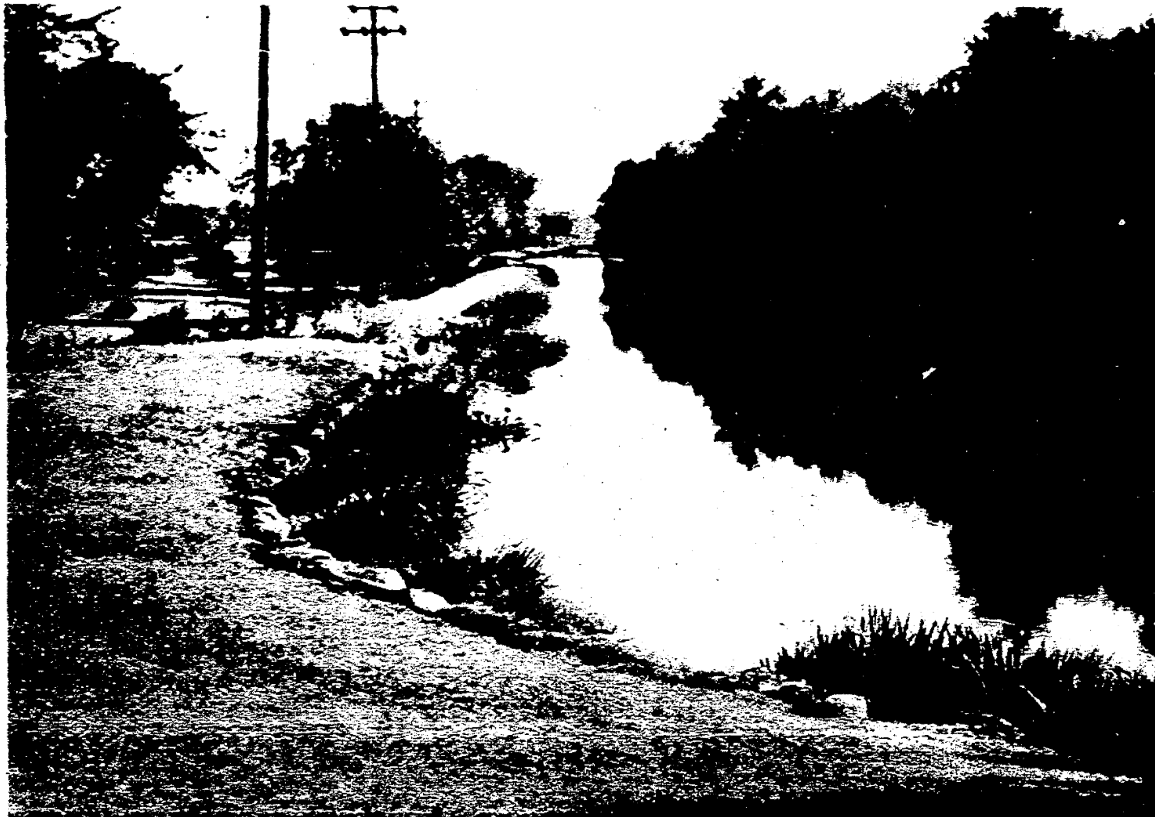
STILL WATERS. Looking south along old Blackstone Canal below spillway at junction of Oak Street and Hartford Avenue, Uxbridge, today. Here, as at many places, rough stones protected bank against the wash.
