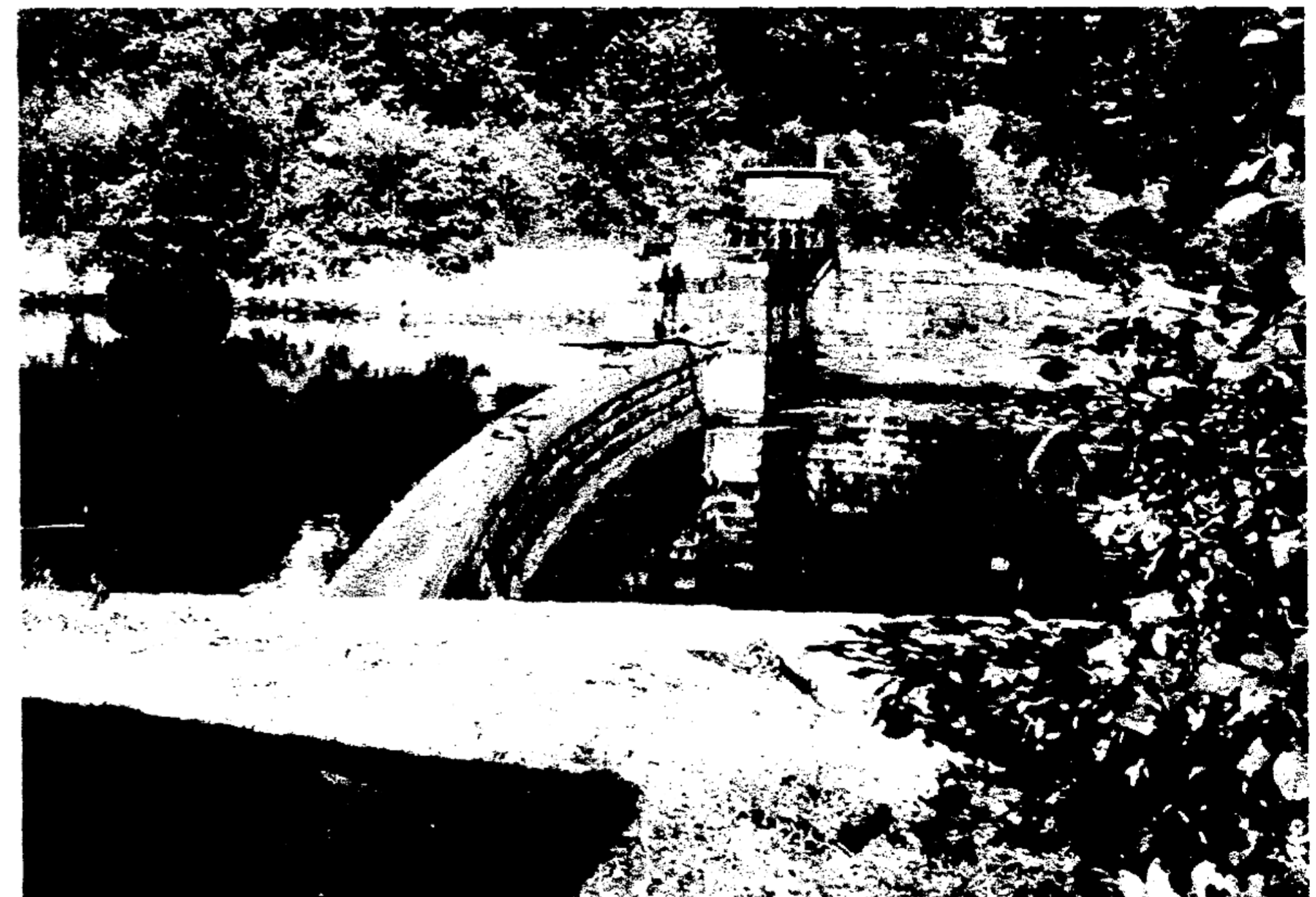
CUT STONE DAM near Ashton (once called "Sinking Fund") built to hold Blackstone at height of Ash-ton-Lonsdale level of canal. Such diversions of water power caused clashes of canal and mill interests.
