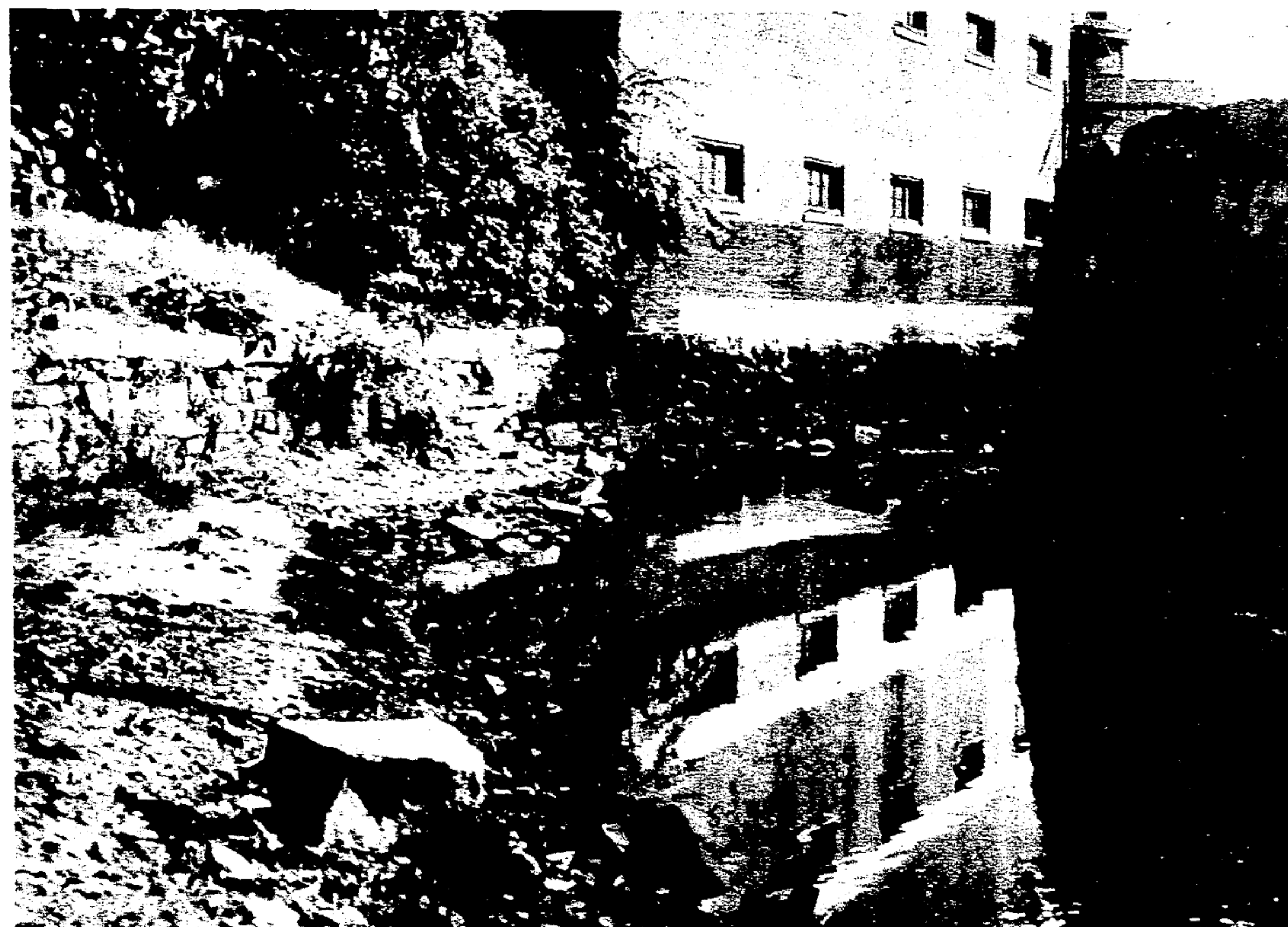
NEAR WORCESTER TERMINUS canal has been mostly covered over and used for storm sewer. Walls of Blackstone waterway still show at end of street called Keefe Place. Michigan lumber once passed this way.
