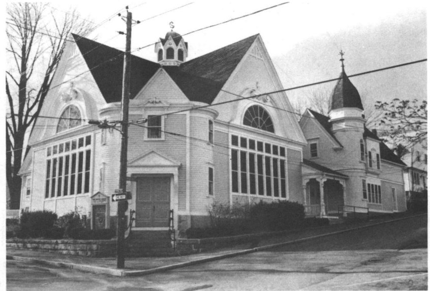
Fig. 29: First Baptist Church (1884), 35 Peirce Street
