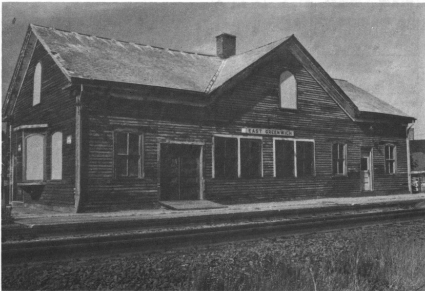
Fig. 28: East Greenwich Railroad Station (1870), 146 Duke Street
