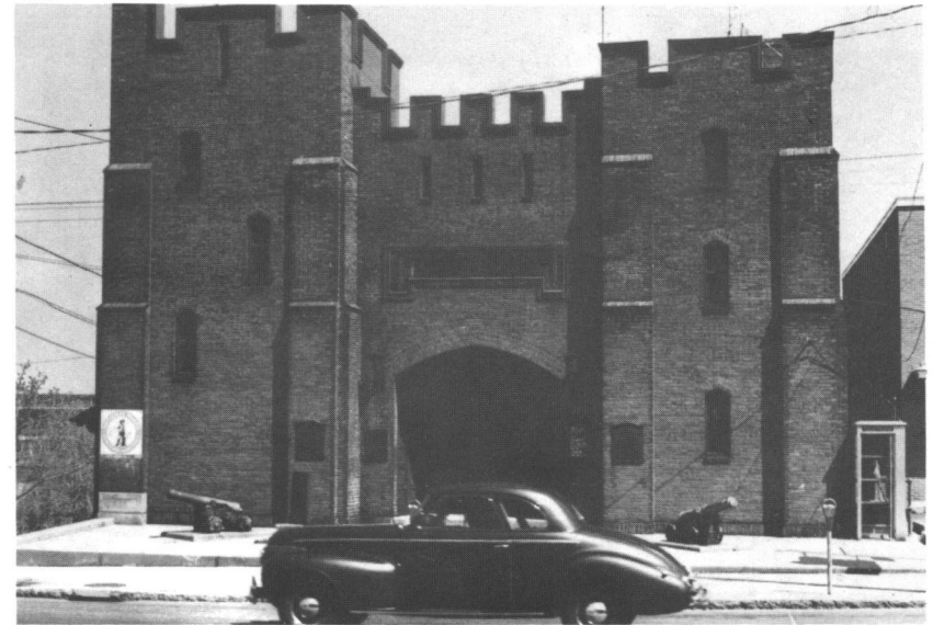
Fig. 34: Varnum Memorial Armory (1914), 6 Main Street
