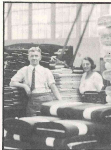
The double and roll section, Plant C of the Sayles Finishing Plants
