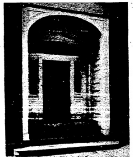
ARCHITECT John H. Cady, who was in charge of the Market House restoration, designed this new doorway on the easterly side after entrance to the John Brown House on Power Street. Both buildings had the same architect.
