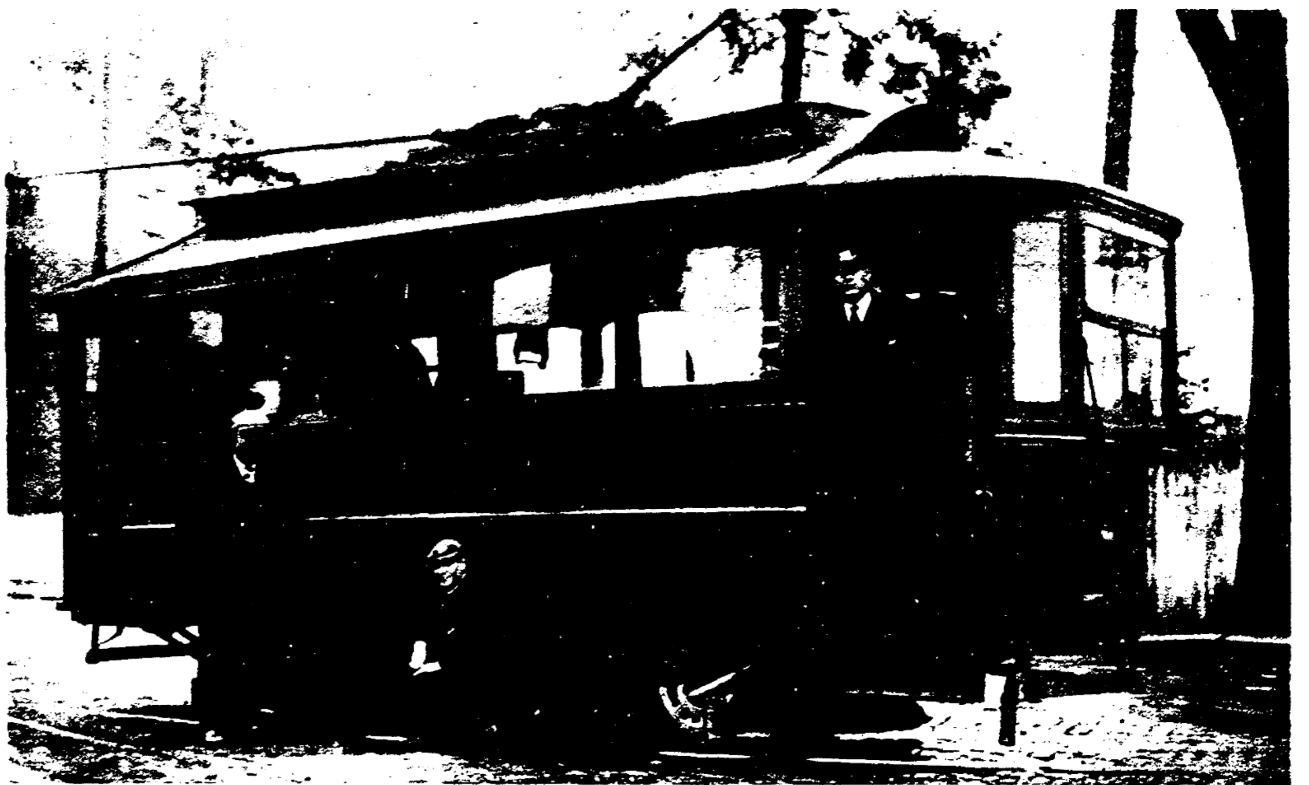
THIS HISTORIC HORSECAR survived into the electric era and had a long and useful life of service, first as pay car, later as official "grinder car" of the United Electric Railways Company, always as "Old 1500."
