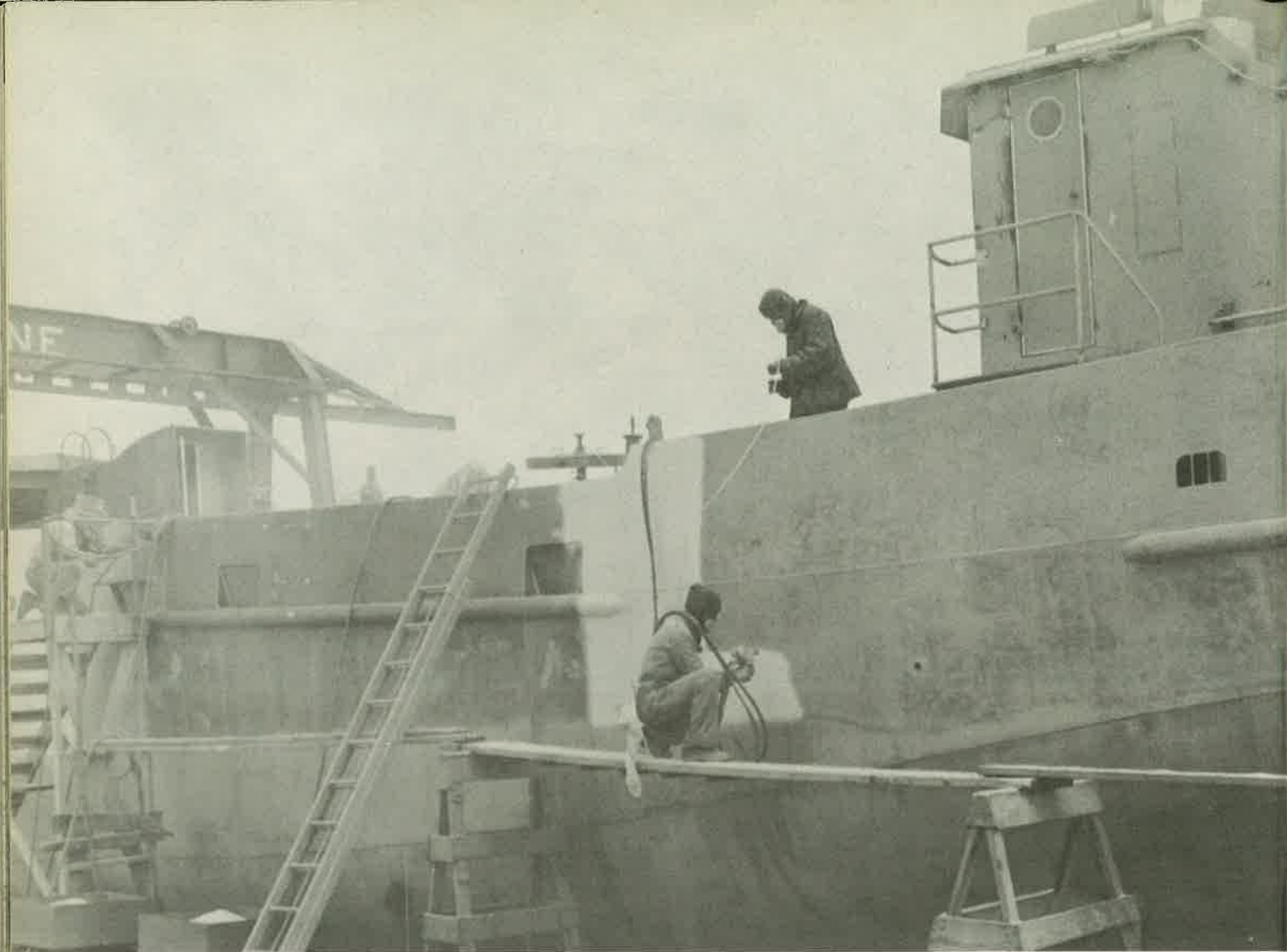
Blount builders apply zinc metallizing to the dragger Cap'n Bill III. Surface is sandblasted to bare steel, and hot zinc is sprayed on, assuring greater resistance to corrosion.
