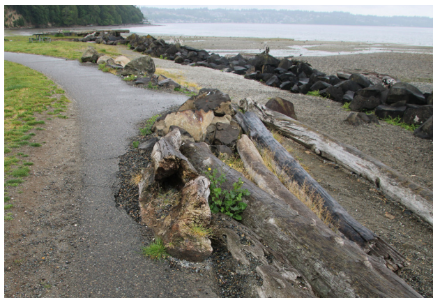
A damaged section of the shoreline trail, with logs pushed up against the pavement.
