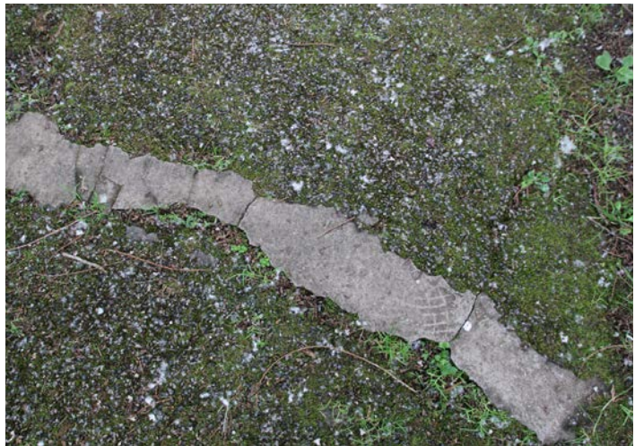
A view of one of the trouble spots in the trail, with eroded pavement and concrete.
