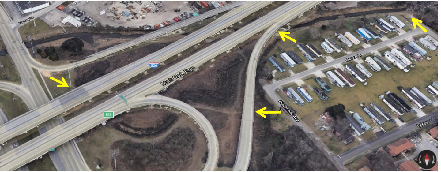
Photograph 3: Foot paths between Ferndale and Rivers Avenue SOURCE: Google Aerial
