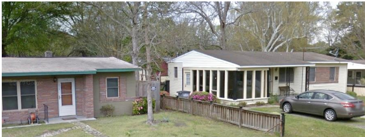
Photograph 19: Example of two types of ranch style homes in the Brentwood neighborhood SOURCE: Google Street View.
