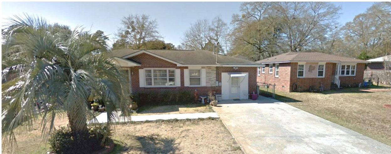
Photograph 6: Standard housing example in the Area 1 neighborhoods SOURCE: Google Street View.
