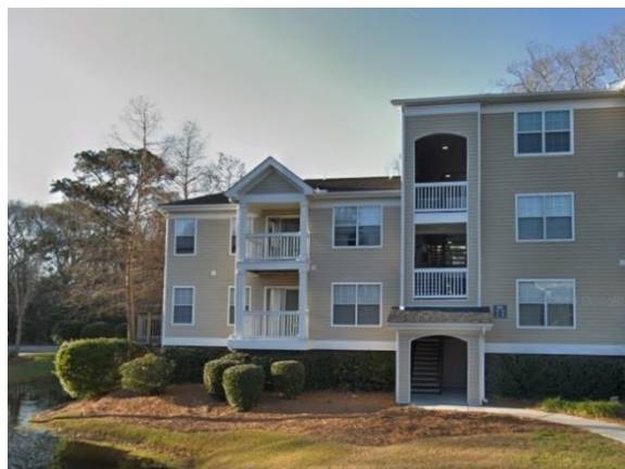
Photograph 27: Radius at West Ashley SOURCE: Google Street View
