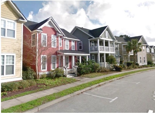
Photograph 9: Example of multi-story, single-family homes being built in Oak Terrace Preserve SOURCE: Google Street View.
