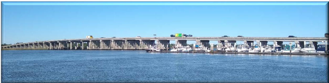
General William C. Westmoreland Bridge over the Ashley River.
