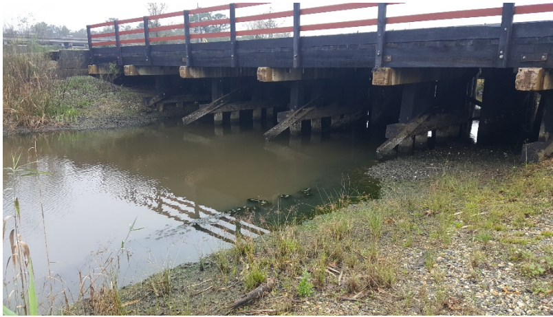
CSX railroad causeway and bridge. (Photo by Three Oaks Engineering)
