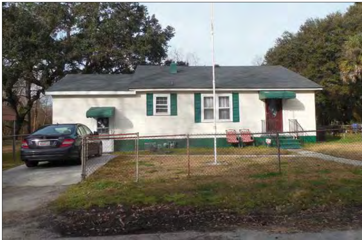
Figure 3.11 View of Resource 1900.01, facing west.
