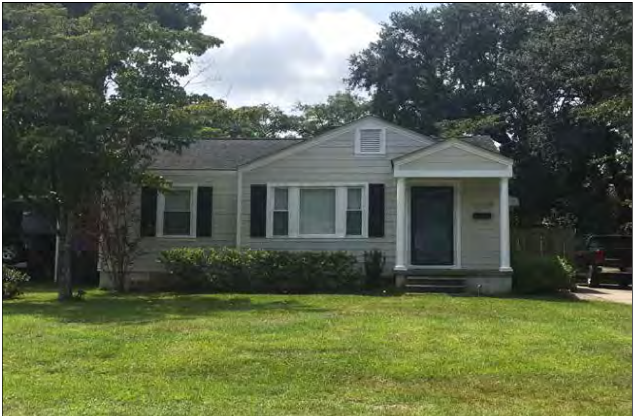
Figure 3.17 Front elevation of Minimal Traditional at 1177 Camden Street (7815.02), showing neighborhood-typical alterations: replacement windows and siding and altered front porch.
