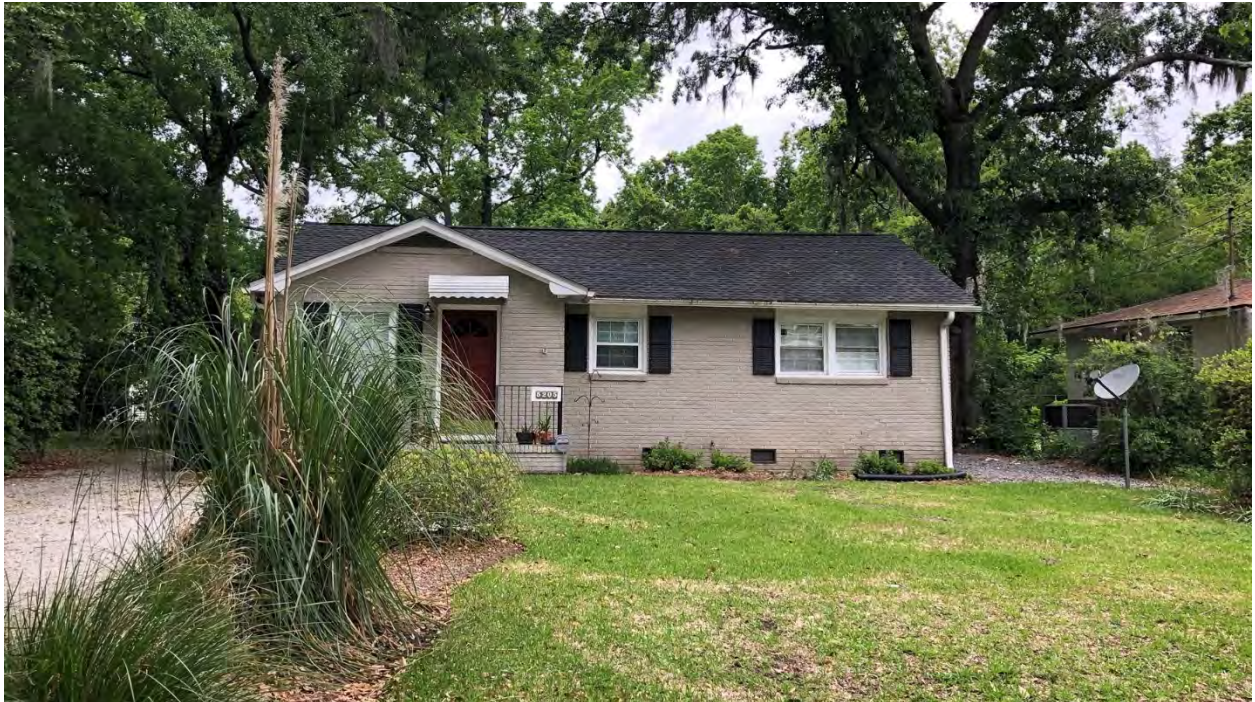
Figure 3.10. East elevation of typical West Cameron Terrace Minimal Traditional house built 1960-1962 (5205 East Dolphin Street).
