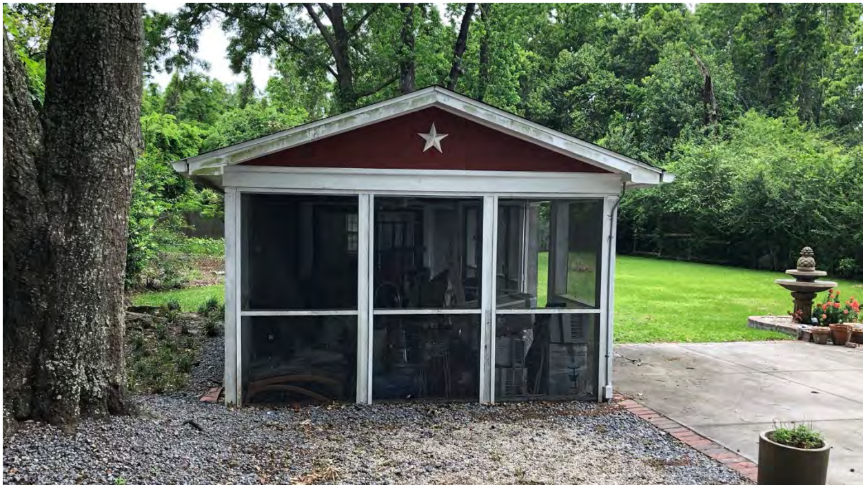
Figure 3.12. Front elevation of typical West Cameron Terrace utility shed (5205 East Dolphin Street).
