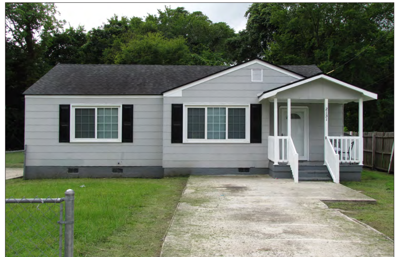
Figure 4.15 Resource 7810.03, an example of a Minimal Traditional house in Liberty Park neighborhood.
