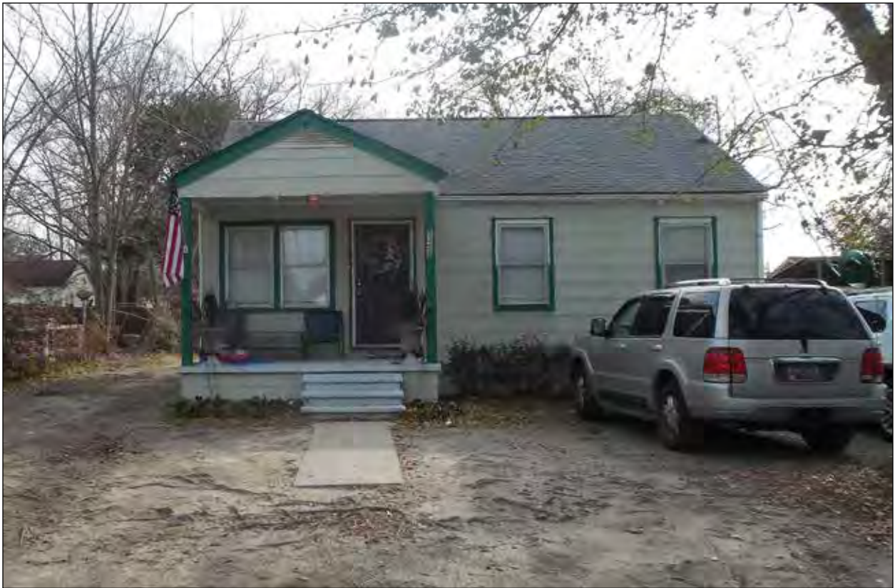
Figure 3.14 View of Resource 1900.04, facing east.
