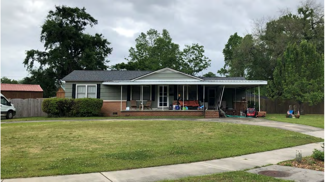
Figure 3.7. North elevation of typical West Cameron Terrace Ranch house built ca. 1958 (5186 Monterrey Street).
