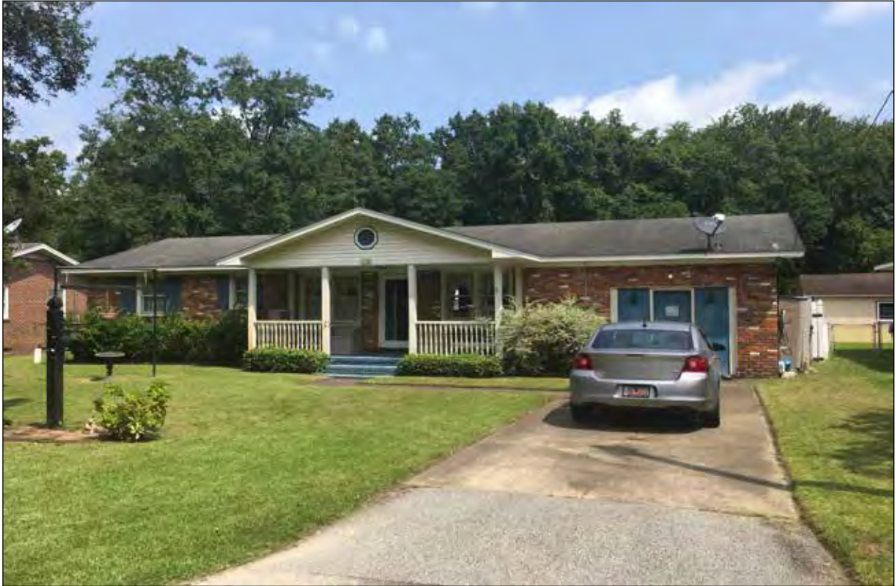
Figure 3.16 Front elevation of Ranch at 1150 Sherwood Street (7815.01), showing neighborhood-typical alterations: enclosed garage, replacement windows, and vinyl siding.
