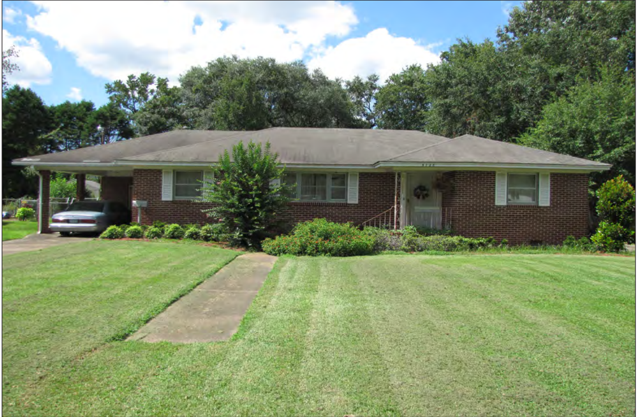
Figure 4.8 Resource 7807.02, an example of a Ranch house in the Cameron Terrace neighborhood.
