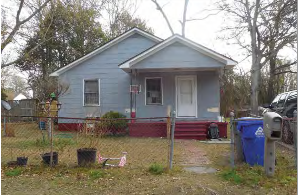
Figure 3.13 View of Resource 1900.03, facing east.
