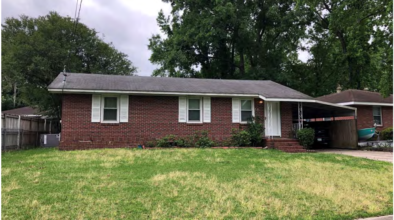
Figure 3.9. North elevation of typical West Cameron Terrace Ranch house built 1960-1967 (1809 Wasp Street) with carport.
