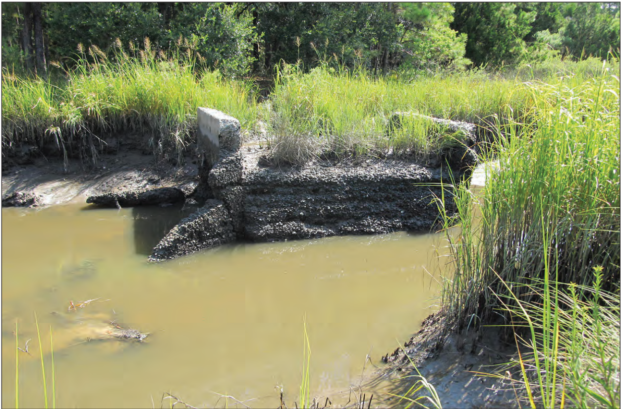
Figure 3.6 Views of concrete bridge portion of 38CH2523: outside of the northern wall, facing south (top); view of bridge from the western side of Bulls Creek, facing northeast (bottom).
