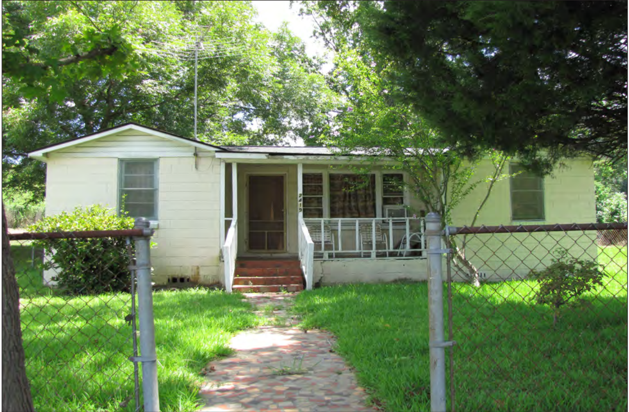
Figure 4.17 Resource 7810.05, an example of a Transitional Ranch house in Liberty Park neighborhood.
