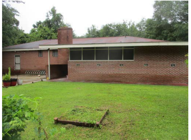
Rear view of subject house.
