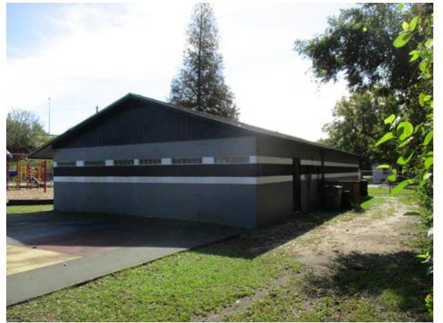
Side/rear view of subject building.
