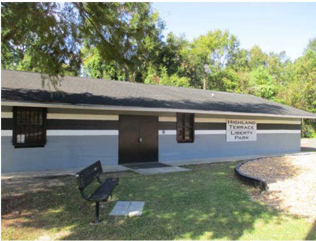
Front view of subject building.
