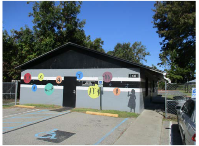
Side view of subject building from parking lot.
