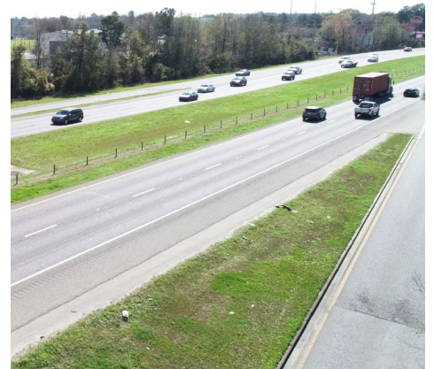
Above: The I-26/I-526 interchange. Below: Free-flowing traffic on I-526 LCC West.
