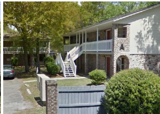
Photograph 31: Etiwan Garden Apartments SOURCE: Google Street View
