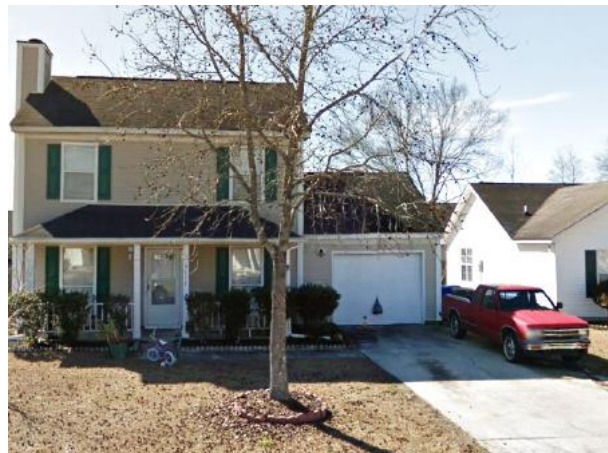
Photograph 13: Single-family house that is characteristic of those in the Area 6 neighborhoods SOURCE: Google Street View.
