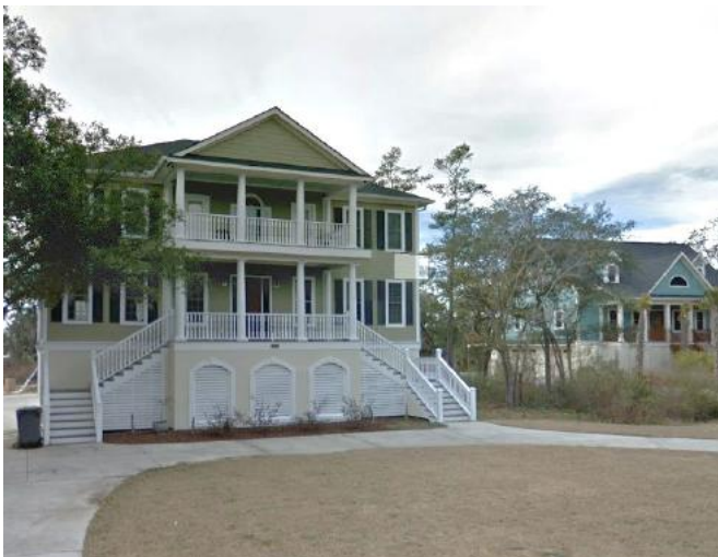
Photograph 14: Single-family house on the Ashley River SOURCE: Google Street View.
