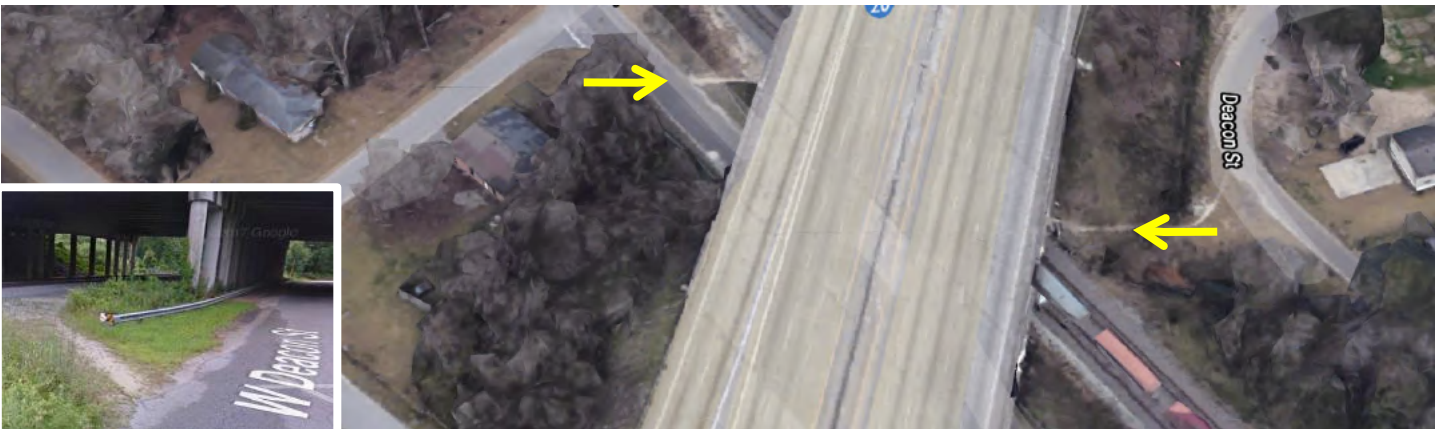
Photograph 5: Foot paths across double-track railroad under I-26 between Highland Terrace Drive/Lacrosse Road and Deacon Street
