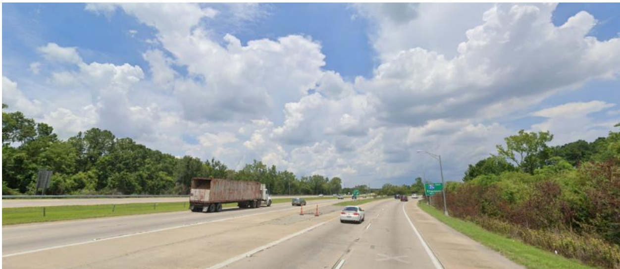
View from I-526 facing north towards the I-26/I-526 interchange.
