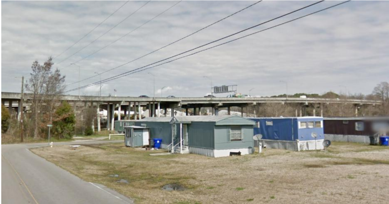
View from the Ferndale neighborhood facing towards I-526.
