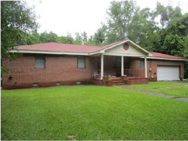
Front view of subject house.
