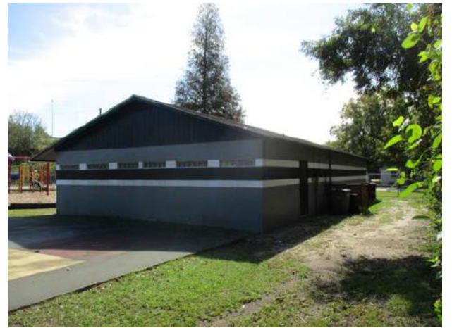
Side/rear view of subject building.
