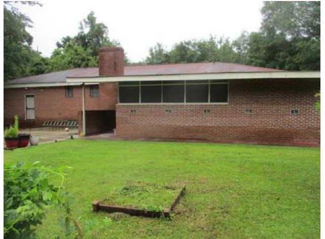
Rear view of subject house.
