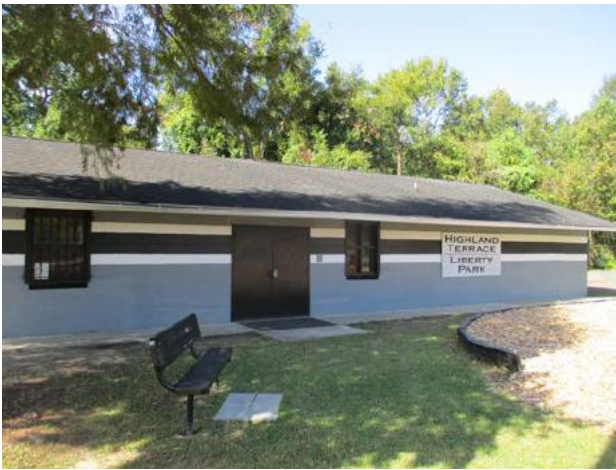
Front view of subject building.
