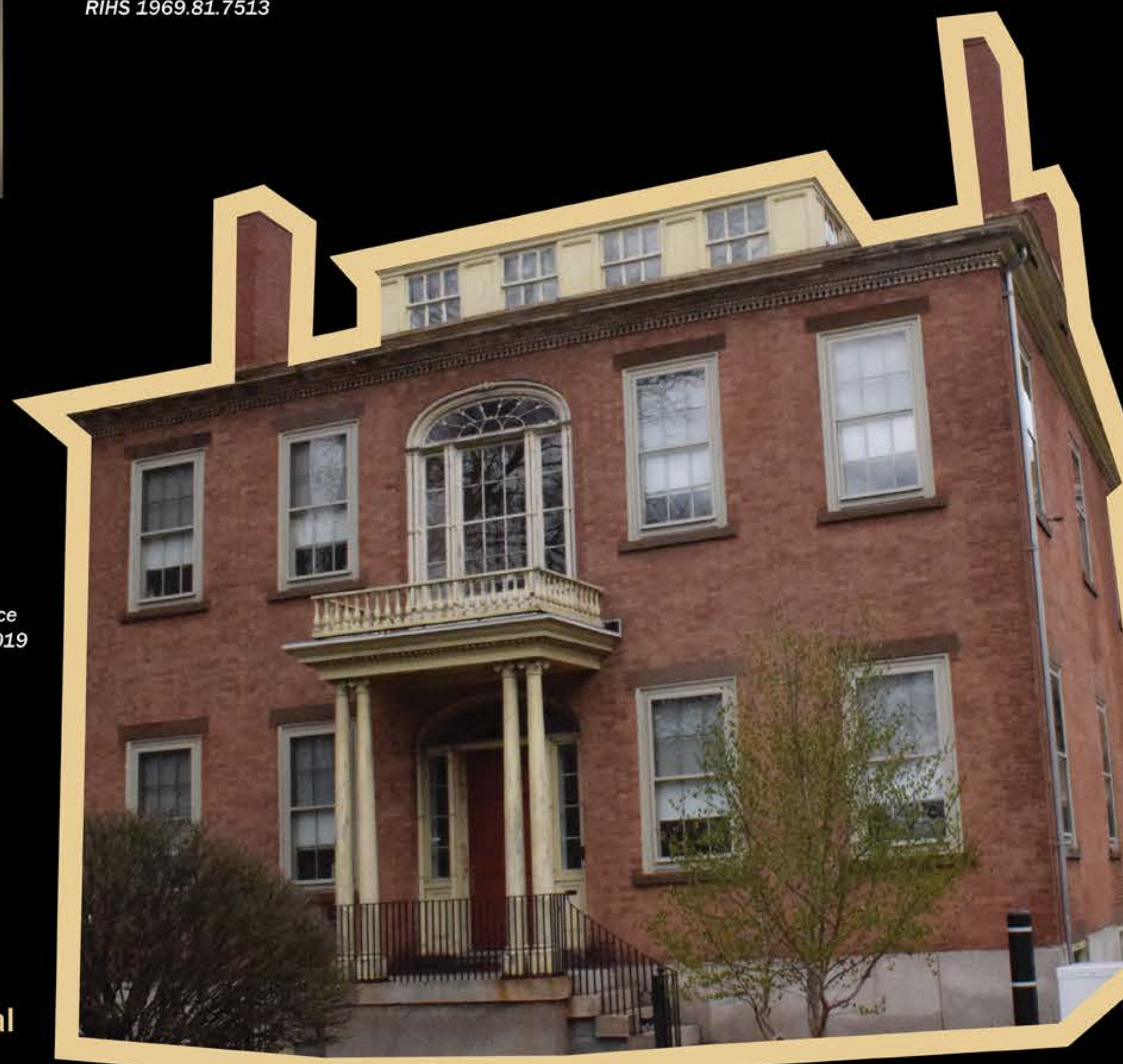
CURE/CORE Office, 33 Chestnut Street, Providence. Courtesy of The Public Archaeology Laboratory, Inc.
