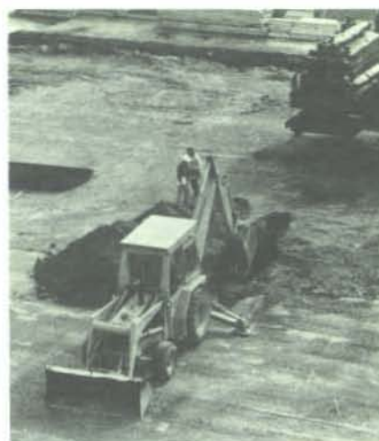
Figure 21. Excavation of the asphalt surface and upper fill deposits was assisted by a backhoe. Photograph by John Miller. Courtesy of Old Stone Square Associates.
