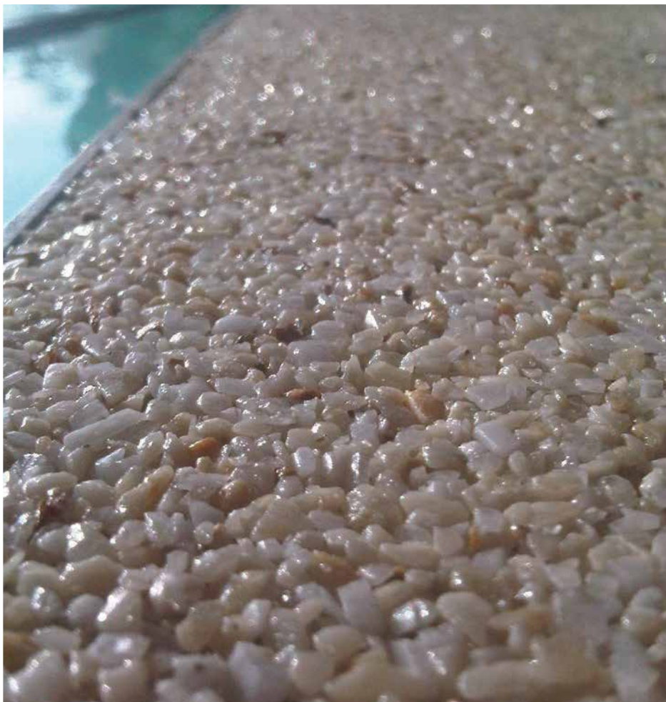
Patterns are created by first preparing the design with Africote's formable 6 mm aluminium trim which is fixed to the floor then placing the various stone colour in each compartment!
